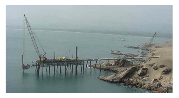
Steel pipe used for piling will be new and unused material only with the yield strength, toughness values and wall thickness selected to suit the detailed final design for the structural system. The chemical and physical properties of each pipe will be recorded and maintained in the as-built record.
