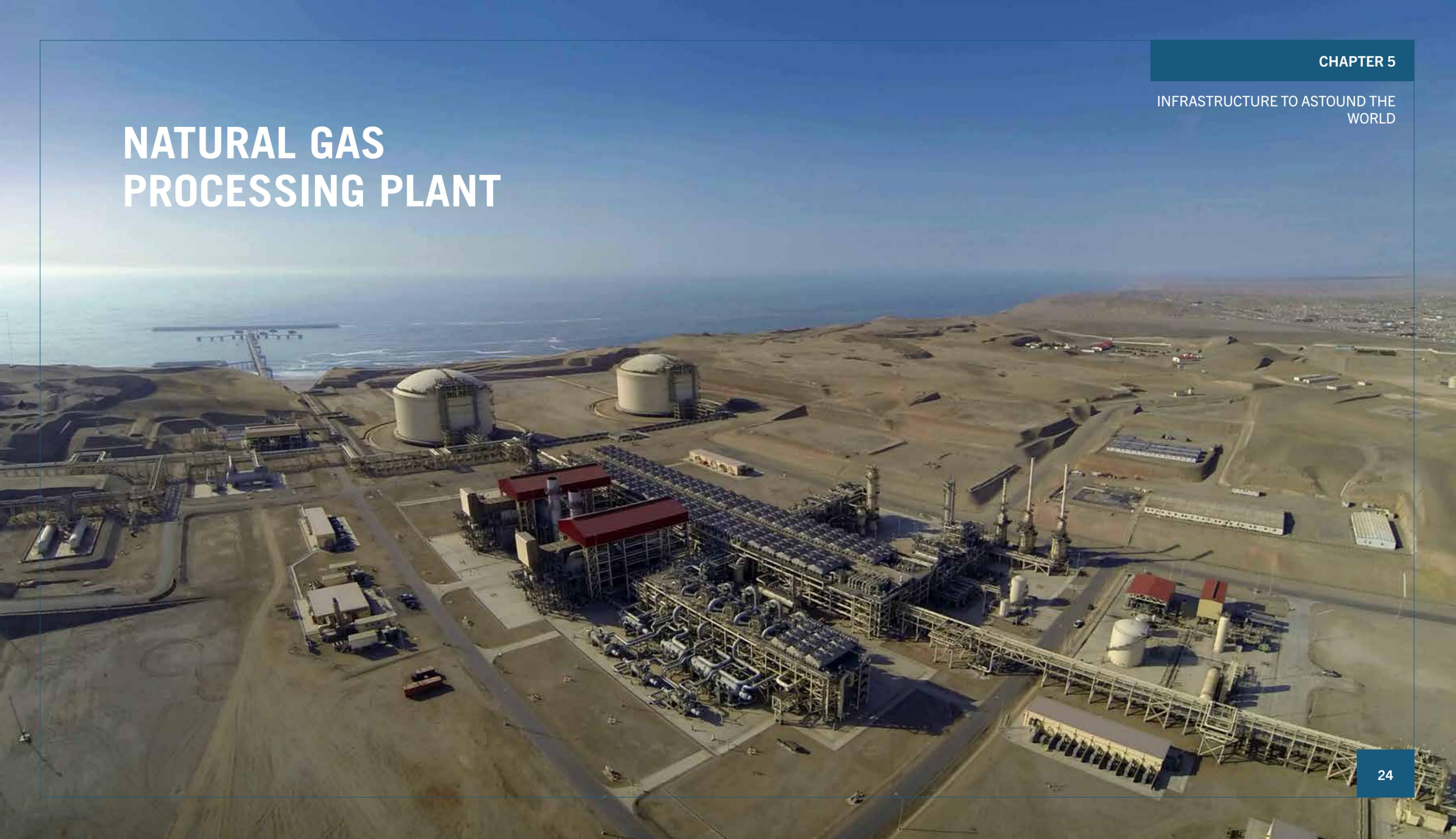
The PERU LNG plant transforms natural gas into liquid to facilitate transport. This is the first liquefaction plant in South America and was built on 521 hectares of land, 163 kilometres south of Lima on the Southern Pan-American Highway.
